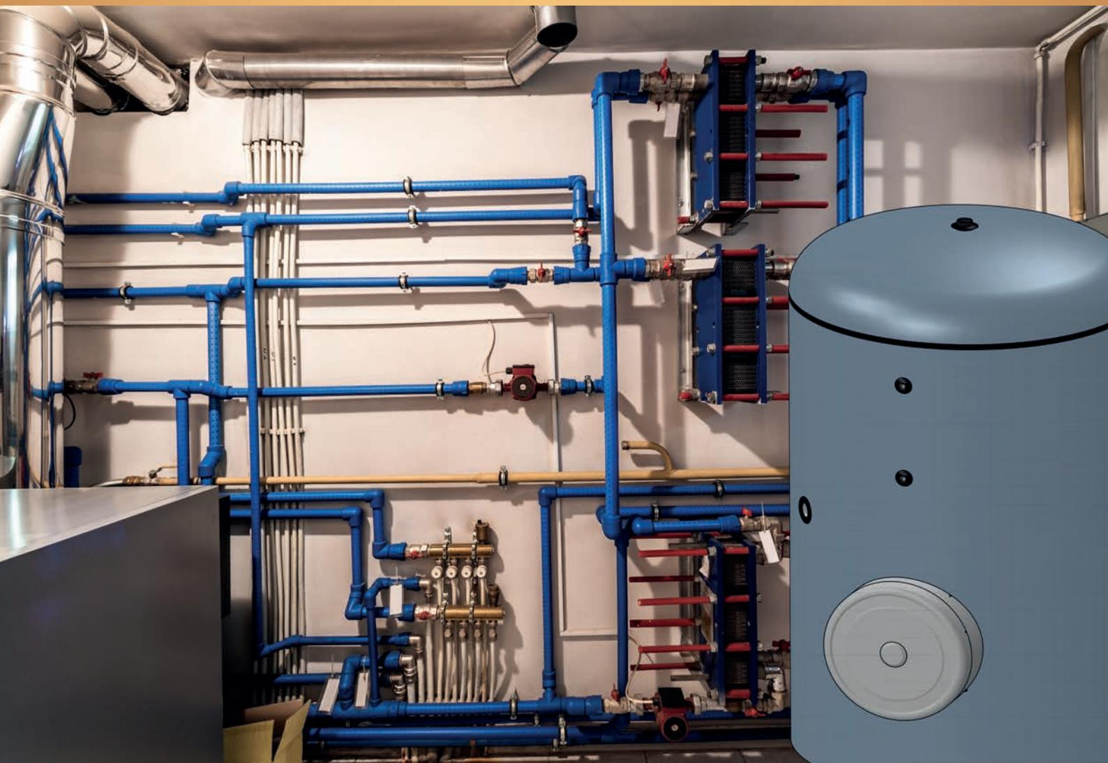
The BVE-WW series tanks are specially designed for primary circuit solar systems. They are equipped with two heat exchangers.
