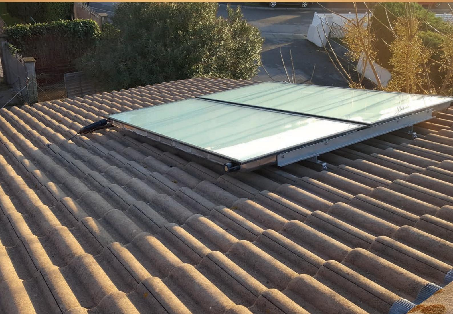
The drain back solar water heater is a self-draining individual solar water heater with a special control station and an intermediate tank.
