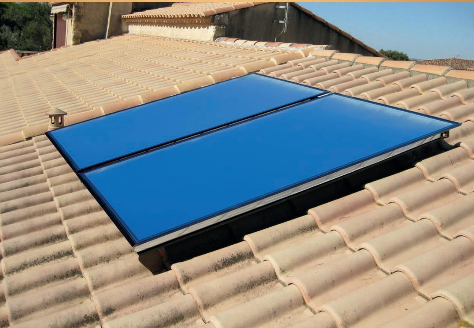
The individual solar water heater consists of one or more collectors, a storage tank and a regulation. The number of the collectors depends on the geographical area and the number of people living in the home. The storage tank can be supplied with back-up energy through an electric resistance, a heat pump or other boilers (gas, oil, wood).
