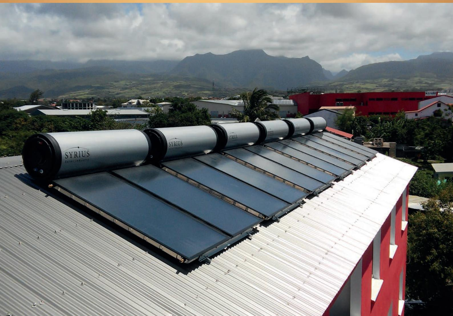
The solar water heater thermosiphon is composed of one or more solar collectors and a hot water tank positioned horizontally, above the collectors, on the roof. The thermosiphon system doesn't need regulation or pump. The circulation of water is carried out alone, by thermosiphon system: hot water, lighter, rises and is stored in the horizontal tank. Cold water, heavier, goes down at the bottom of the tank and of the collector.
